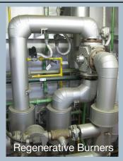
Regenerative burners help lower combustion energy requirements by about 11% per year.
